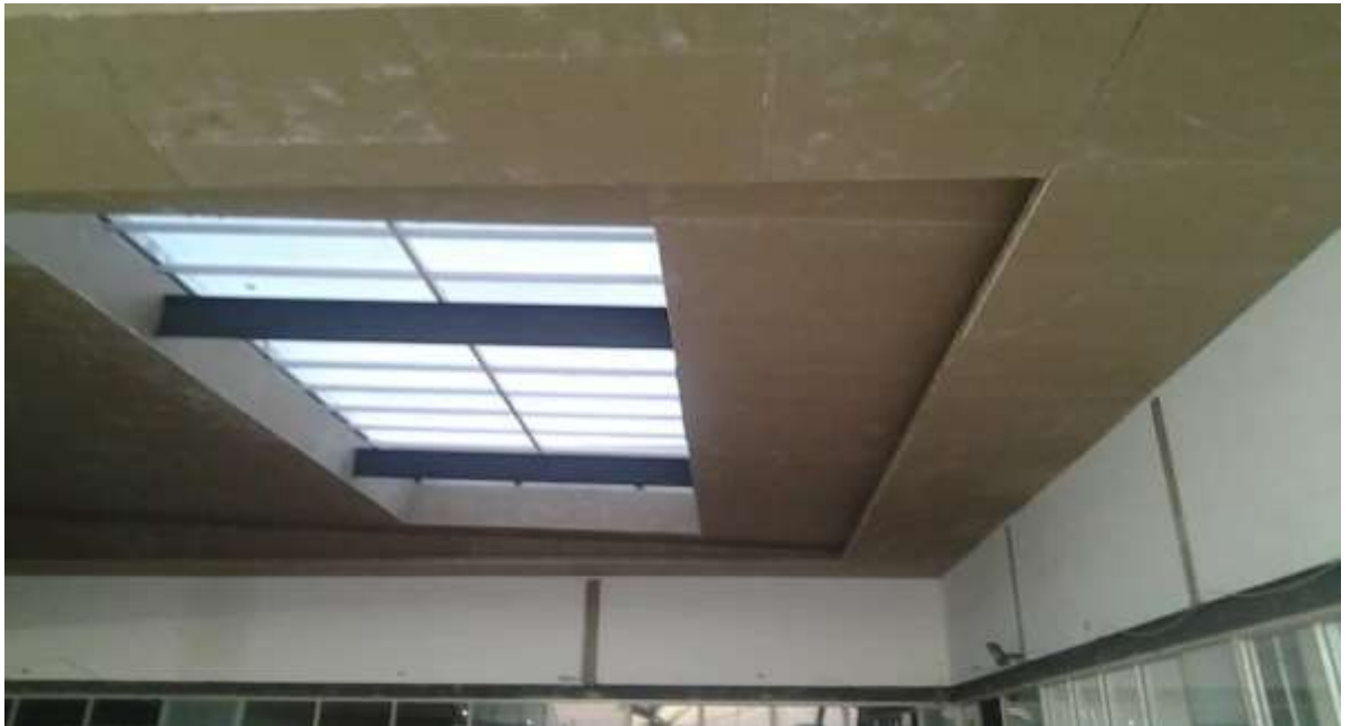
CEILING INSTALLATION WORKS
