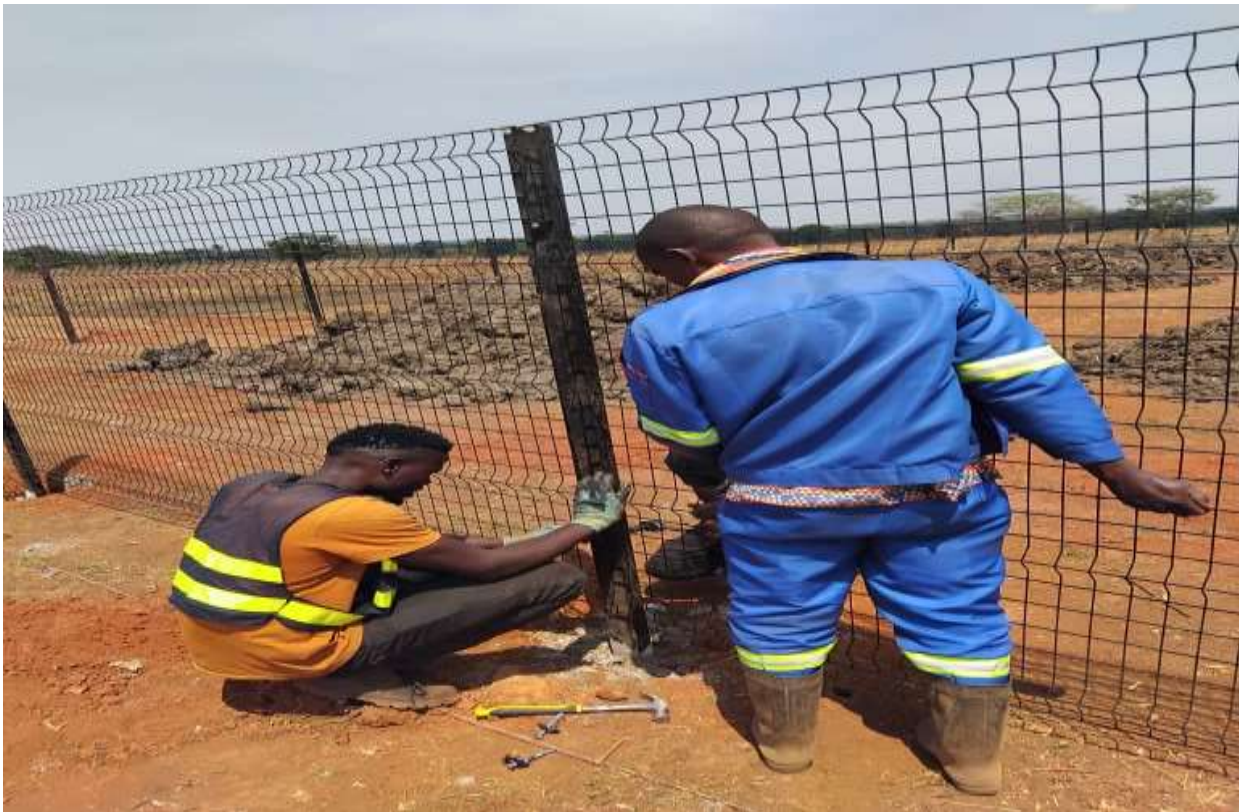
HIGH VISIBILITY FENCING
