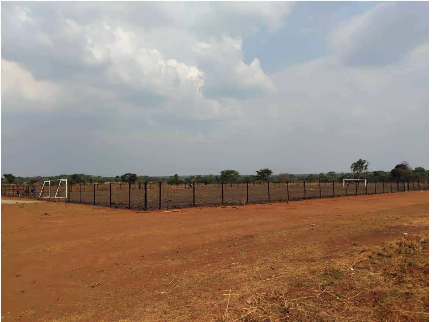
CONSTRUCTION OF A FOOTBALL PITCH
